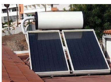
Fig. 12.3 Solar flat plate collector
