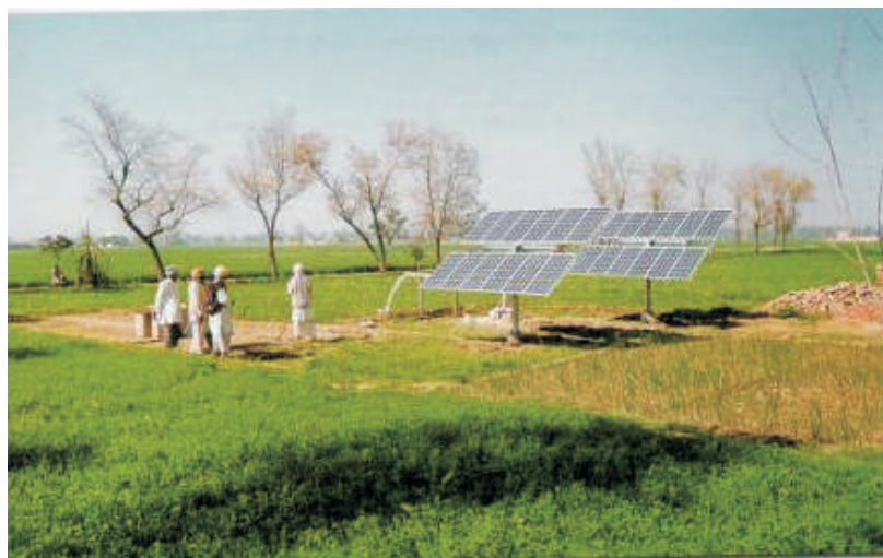
Fig. 12.2 Photovoltaic Water Pumping
